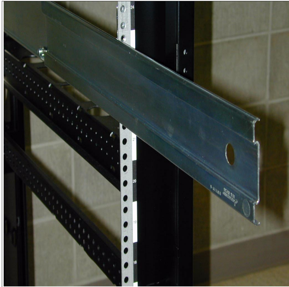
Figure 3-15 Rail in locked position
